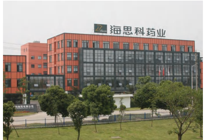
Chengdu Haisco Operation Headquarters and R&D Center
